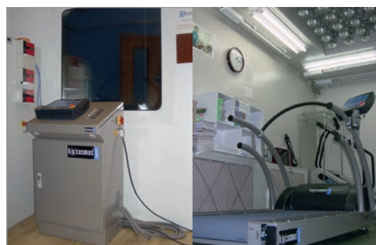
environmental chamber installation with remote control
